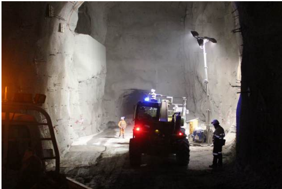
Figure 11: Shotcrete application Cadia East mine, NSW Australia.
