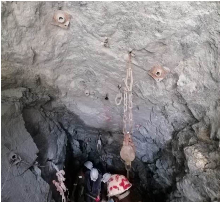
Figure 2: Example of Split Set Installation in Winze
