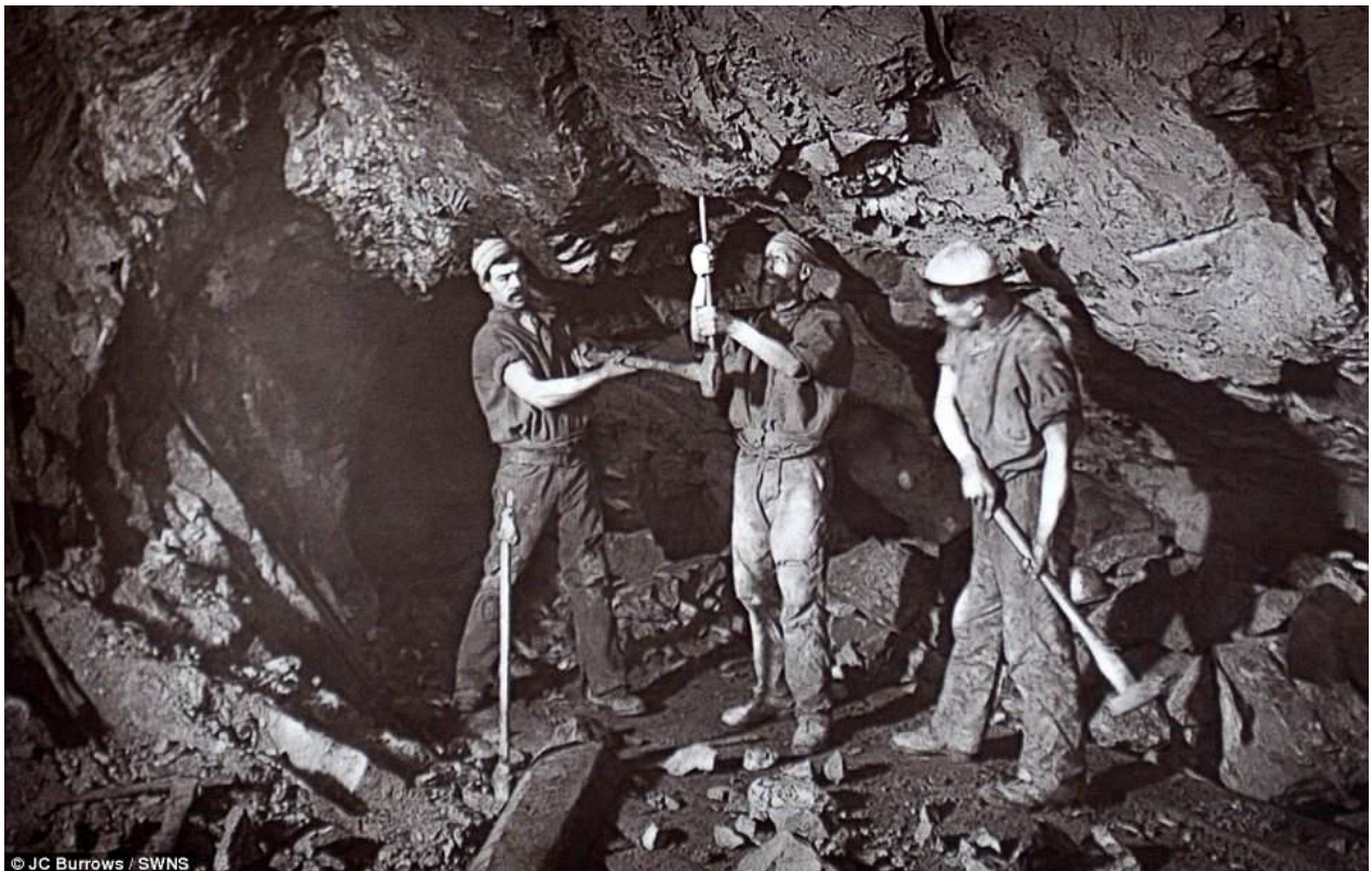
Figure 4: Beating the bore - drilling by hand (photo JC Burrows: East Pool Mine Cornwall, UK 1890).
