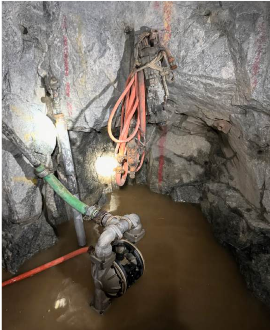
Figure 6: Dewatering the winze with the pneumatic double diaphragm pump
